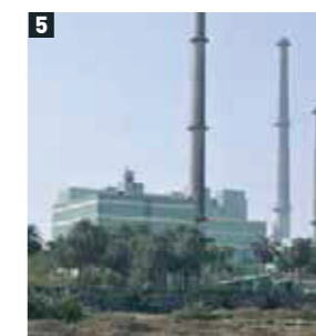
5 India's first Power Reactor Fuel Reprocessing plant (PREFRE) and Advanced Fuel Fabrication Facility (AFFF) at Tarapur.
